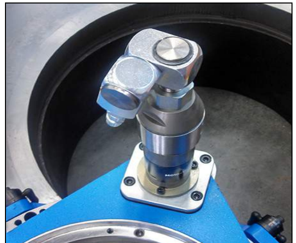
FIGURE 3-25. MOTOR INSTALLED (FF1200 SHOWN)
